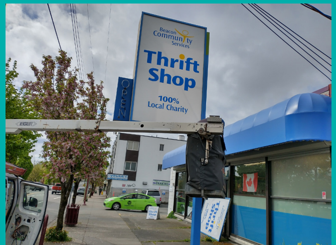
Installing the sign at the new Quadra Street store
